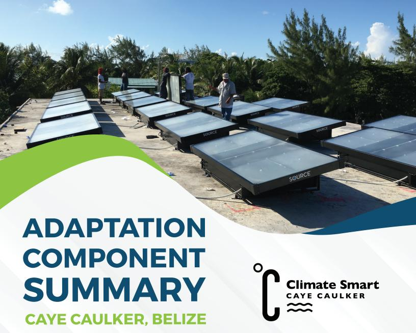
In 2019, the Inter-American Development Bank with the assistance of Environmental Resources Management (ERM), officially launched its first climate change adaptation pilot project to provide an independent and off-the-grid water production system for the island of Caye Caulker. A hydropanel array was installed and commissioned at both the Caye Caulker Roman Catholic School and Caye Caulker Health Center.
